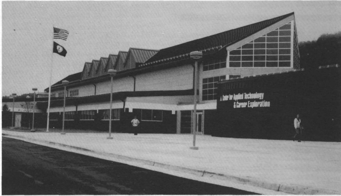
Photo 1. Entrance, Center for Applied Technology and Career Exploration.
