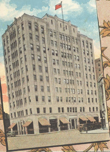
METROPOLITAN BUILDING, WINDSOR.
